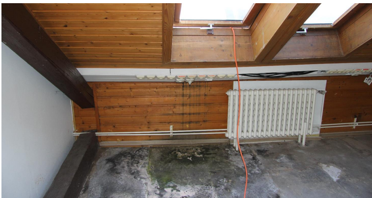
Fig.: 1 Leaking in the loft
