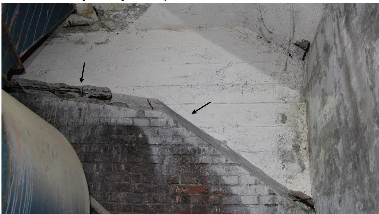
Fig.: 5 View of the ceiling rib – damaged lower reinforcement, cracked cover layer
