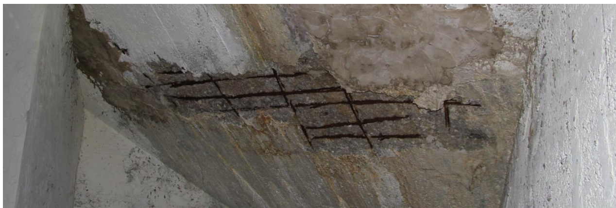
Fig.: 3 Damaged cover layer and corroded reinforcement
