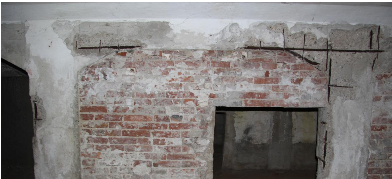
Fig.: 8 Damaged cover layer – it can be re-profiled
