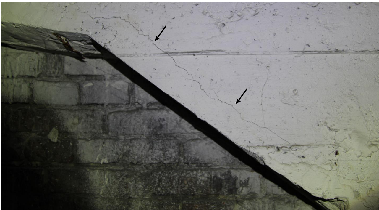
Fig.: 6 View of the ceiling rib – damaged lower reinforcement, cracked cover layer
