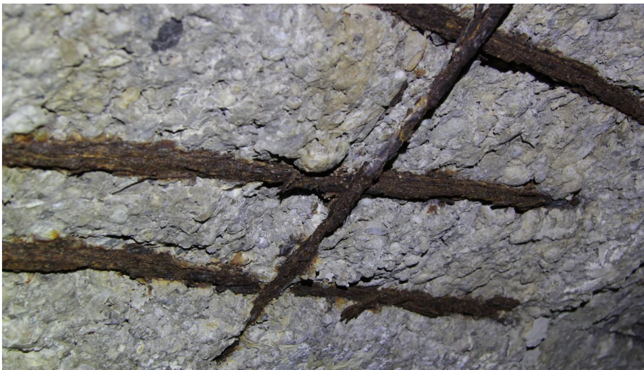
Fig.: 4 Damaged cover layer and detail of the corroded reinforcement
