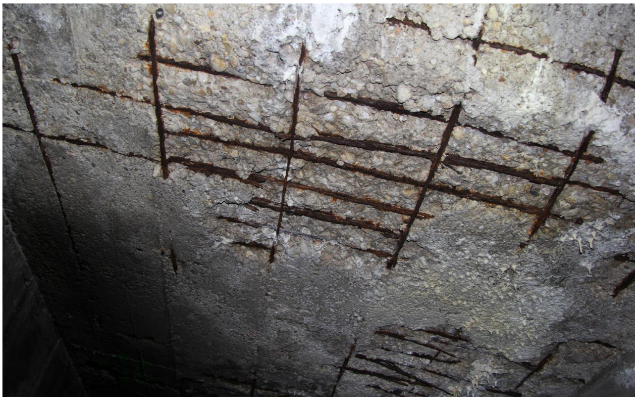
Fig.: 7 Damaged cover layer and detail of the corroded reinforcement
