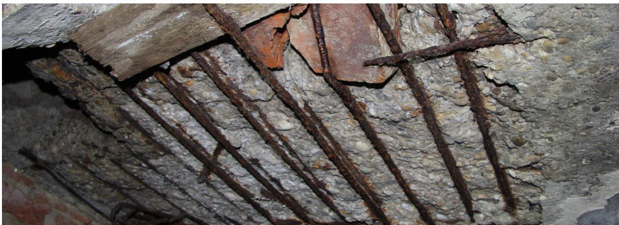
Fig.: Damaged cover layer
