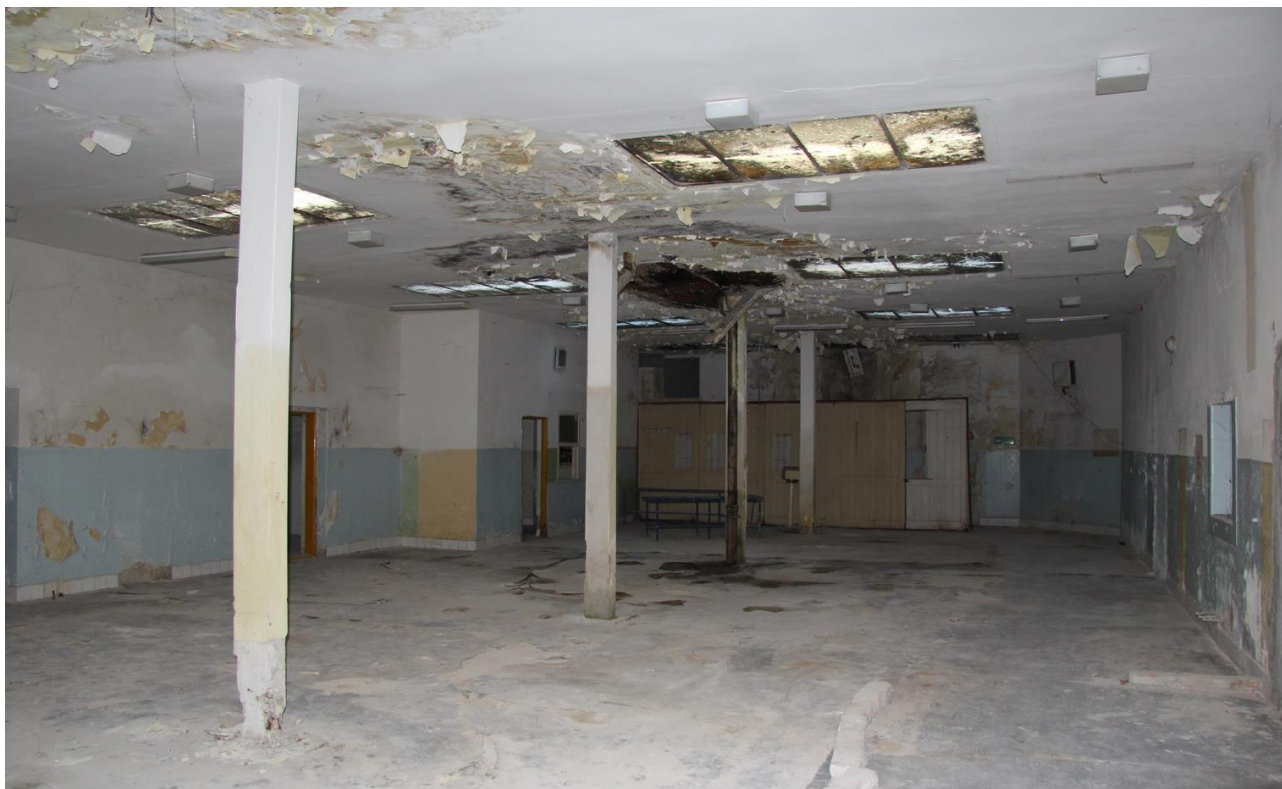
Fig.: 13 Large room in part K – ceiling in a state of serious disrepair
