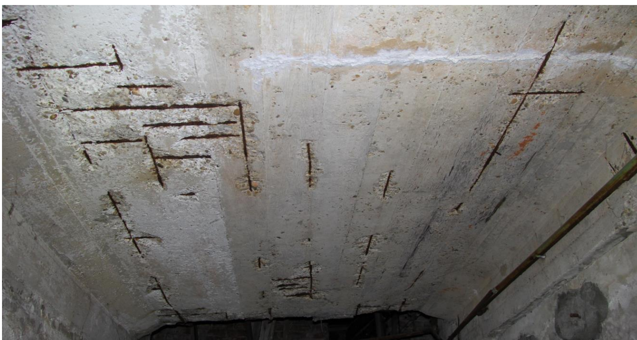
Fig.: 9 Damaged cover layer – it can be re-profiled
